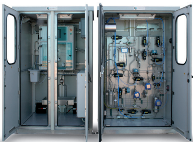
Analyzer shelter with integrated sample preconditioning system
